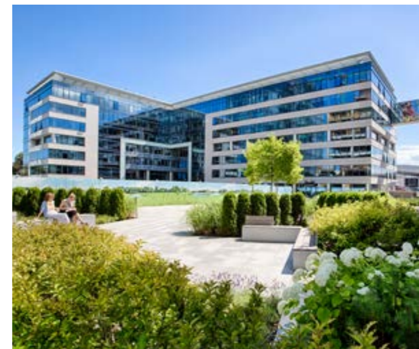
Kompleks Olivia Business Centre, Gdańsk
